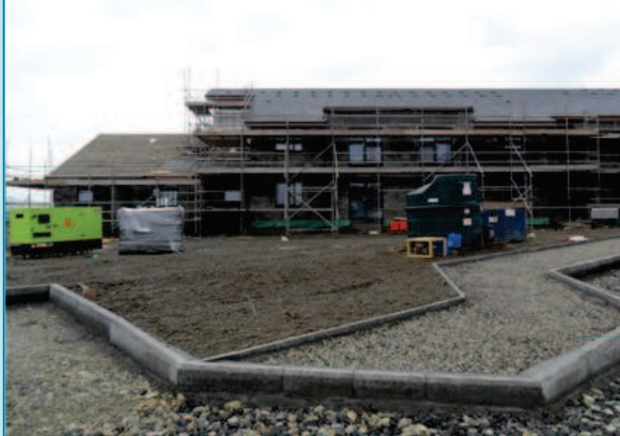
Mull Progressive Care Centre under construction
